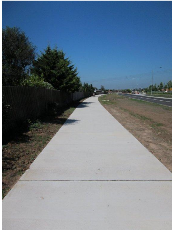
Figure 3. E-Crete Footpath (Calder Freeway Interchange)
